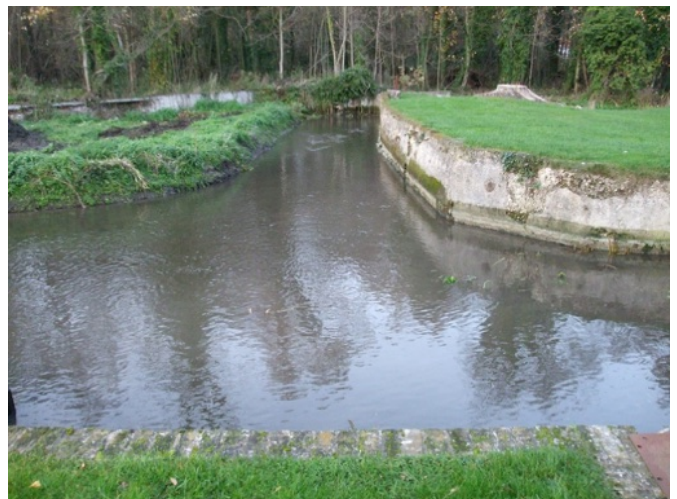
Uxbridge River Stretch cleared of vegetation
