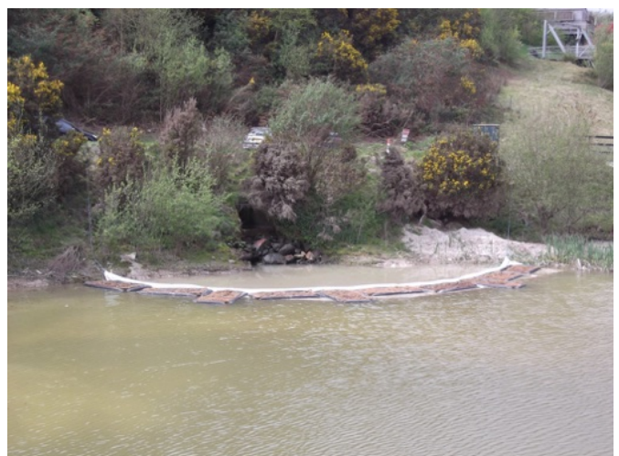
Eden Project planted with a silt curtain and reed rafts
