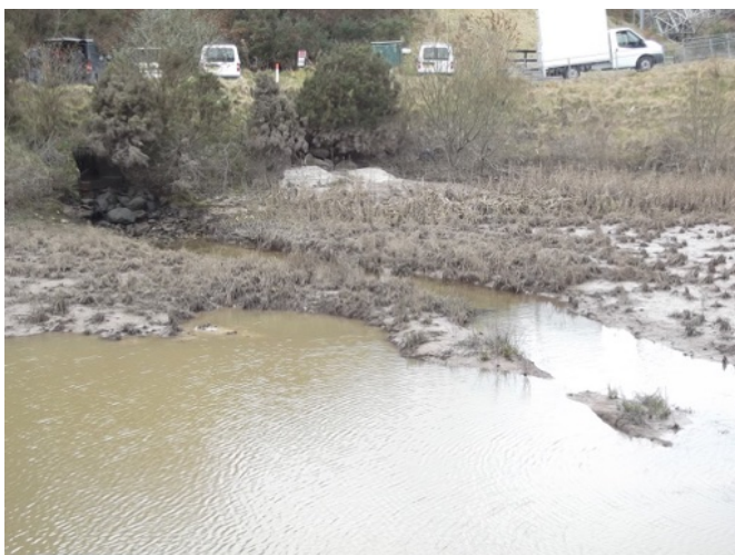
Eden Project flood reduction pond full of silt
