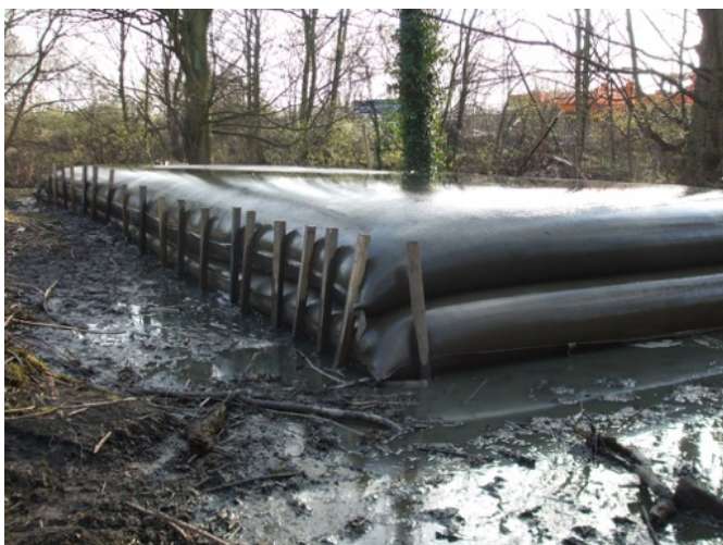
De-watering bags stacked to save space on site
