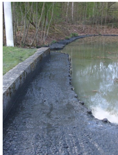
Nicospan area filled with silt removed from the pond
