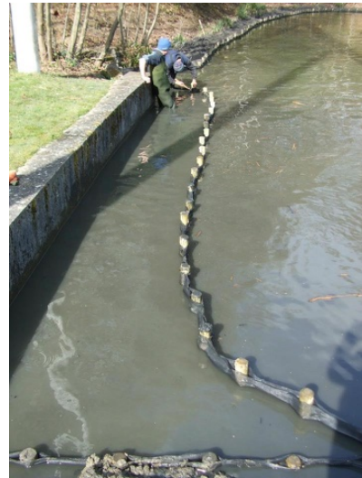
Nicospan area within the waters edge ready for the silt
